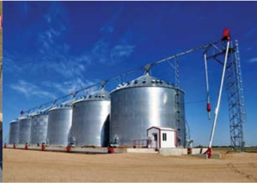
Installation of Grain Pump loop system into existing bin structure.
