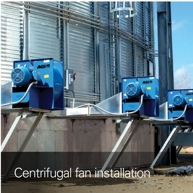
Centrifugal fan with rain hood installation
